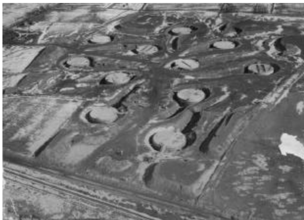
Air Photo, Tank Farm 5 (1943)
